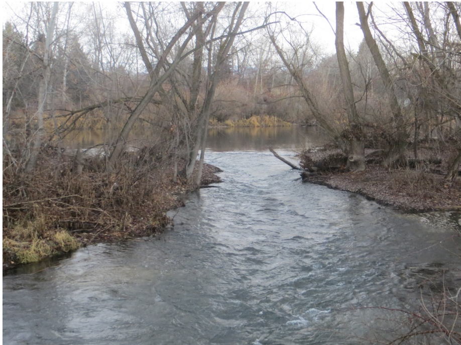
New Dry Creek Diversion Side Channel, December 21, 2018. Q_{\text{Glenwood}} was gaged at 245 cfs, with approximately 150 cfs spilling into the side channel through a bank blow-out that has been developing over the years.
